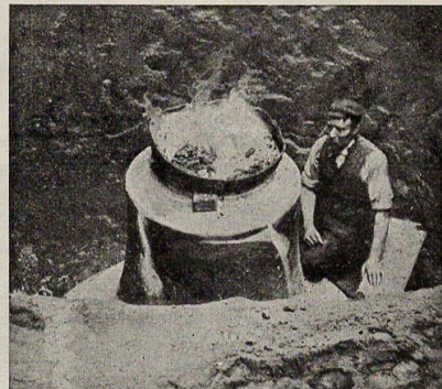
4. Then the core is baked hard or is dried by means of fires lighted on the top, in an iron pan as shown here.
