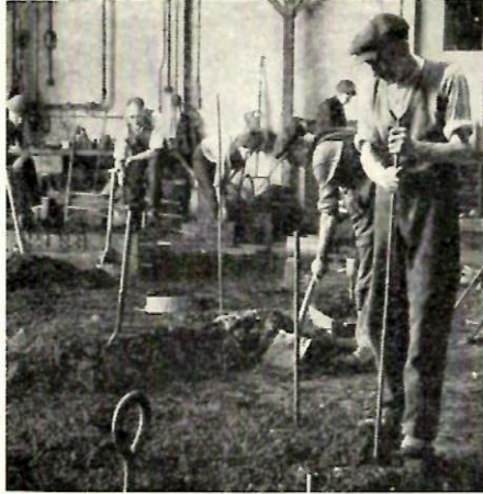
Before a bell can be cast a mould and core must be made from a composition called "foundry loam."
