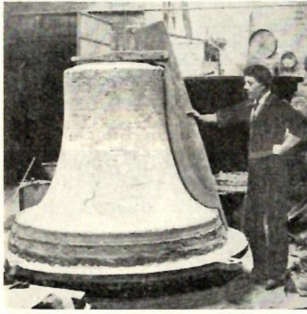
Gradually the core is built up, being modelled by a shaped board that works round the loam core.
