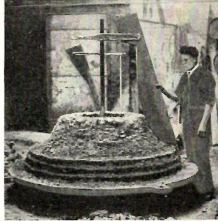
The core, shaped like the inside of a bell, is made from "foundry loam," and here we see the work started.
